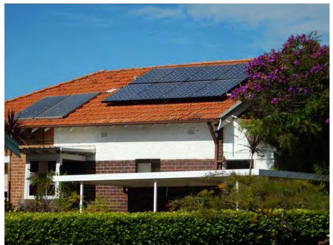
Figure 4.3 - Solar collectors (Photo-Arterra)
